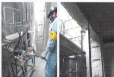
Aseismic reinforce, Brace install, Anchor holes.
